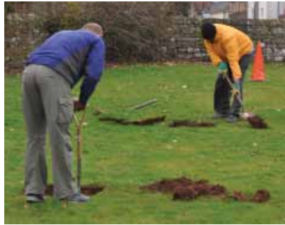
Getting the ground prepared for the goal posts
